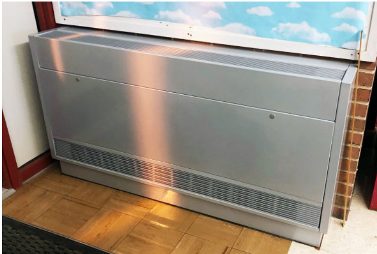
Marley CUH Cabinet Unit Heater (Replaced the Original Unit Heaters)
