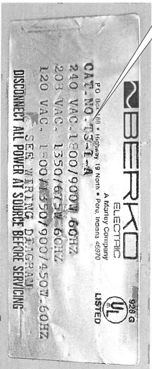
Fig. 5 Berko Nameplate Label (Located Adjacent To Plug And Socket)
